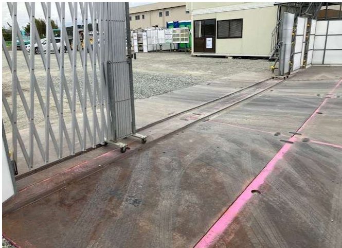
鉄板敷&溶接OK
