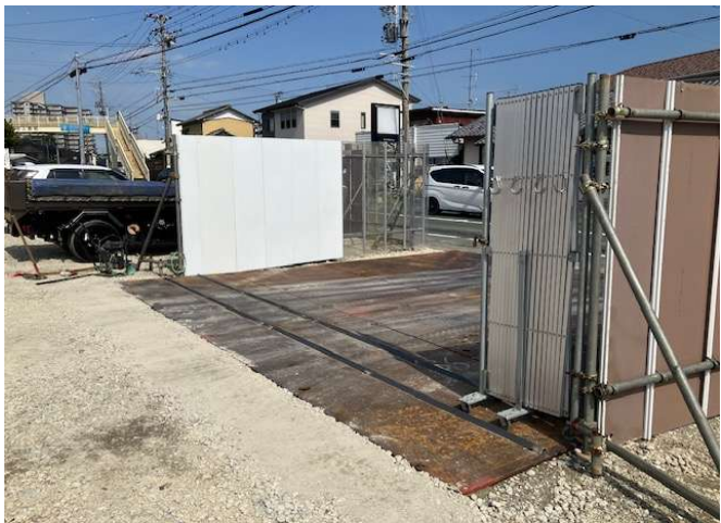
鉄板敷 & 溶接OK
