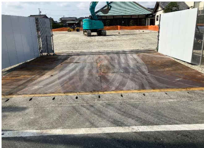
鉄板敷 & 溶接OK
